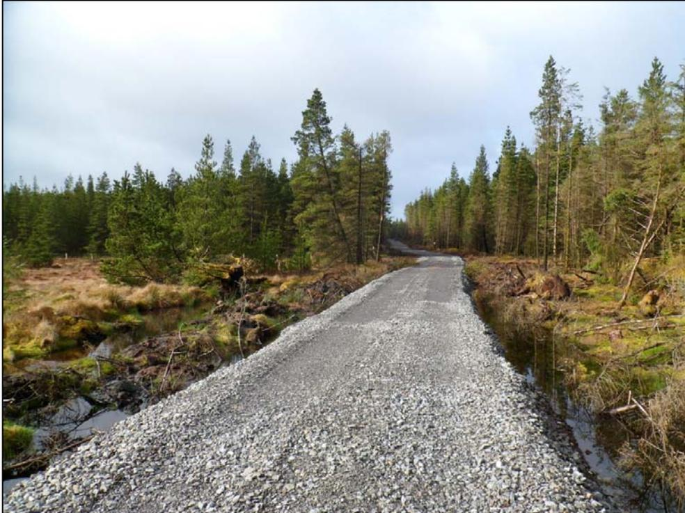
Photo 7 Example of floated access track on site
